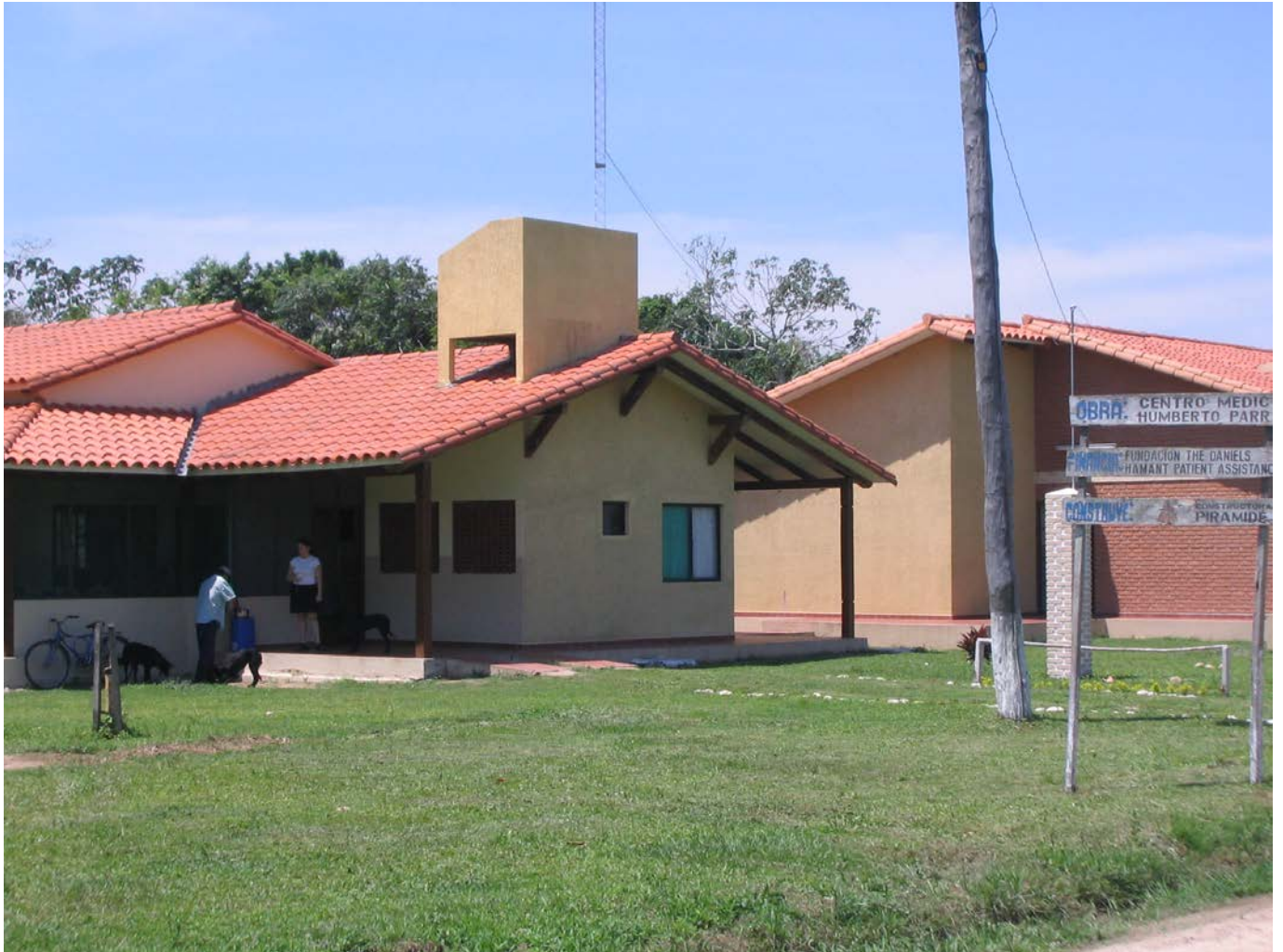
The living quarters for the clinic are located on the left while the clinic building itself is partially seen on the right
